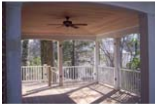
Covered Deck Arlington, VA
