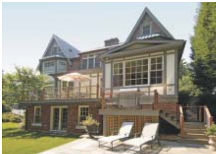
The additions allow for a new breakfast room and playroom, while improving access to the new deck and rear yard.
