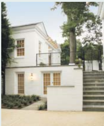
The two-story structure claims unused space for needed storage.
