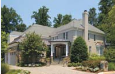
The new entranceway creates warmth and character, while allowing for the added garage space the client desired.
