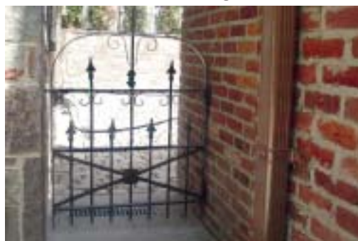
Reclaimed brick and cobblestone and a repurposed iron gate add to the charm of the project while demonstrating the benefits of deconstruction.
