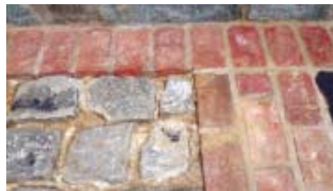
Antique brick and cobblestones recovered from old Georgetown helped to ensure that the new driveway and carriage house blend seamlessly with the existing home.
