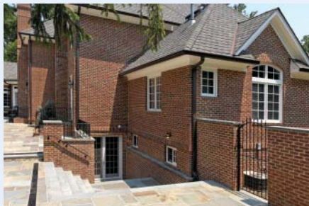
The client wanted a private entrance to his new lower-level home office, which would be appropriate for business associates and seamless to the existing space.
