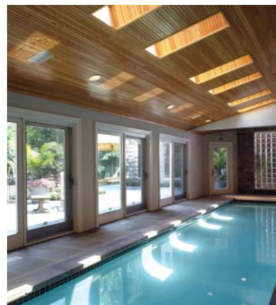
A combination pool heater/dehumidifier unit provided the client a solution that was both energy efficient and effective in controlling moisture for improved air quality.
