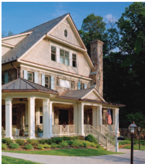
Permeable concrete pavers at driveways and other solid surfaces help to absorb rainfall, which is then released slowly, reducing runoff.
