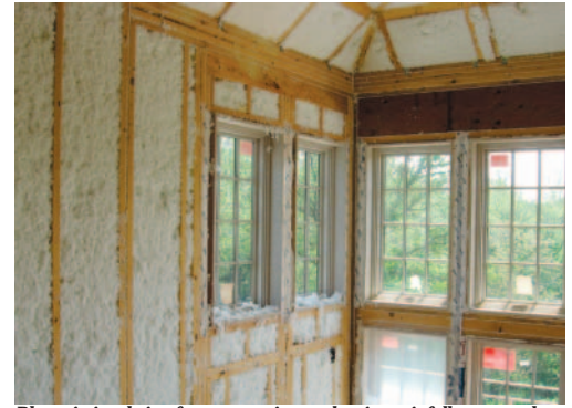
Blown-in insulation forms a continuous barrier as it fully surrounds wires, pipes and other obstructions, and achieves the top "Grade 1" rating for insulation effectiveness.
