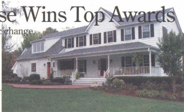
This remodeled farmhouse in Great Falls won two awards.
