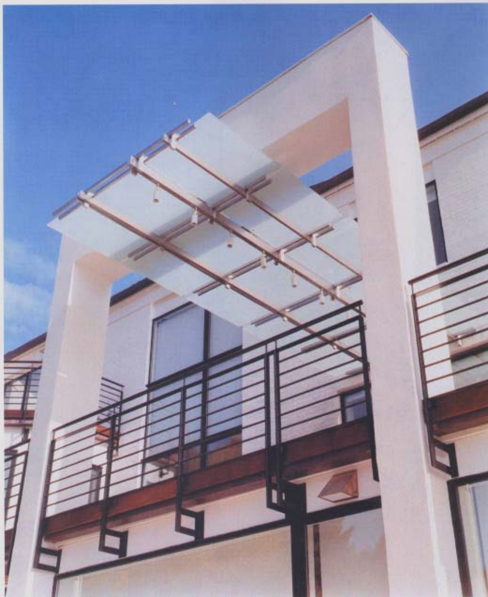
McInturff bridged the barriers between inside and out, forcing a frosted glass ceiling through the exterior wall and creating a dramatic, translucent roof for the balcony (above). He collaborated with Bleam for a unified design incorporating an indoor pool, an outdoor pool and a reflecting pool. The horizontal line formed by a wing housing the indoor pool is interrupted by a reversal in the angle of the roofline as mullions in the tall window create a Mondrian-like grid (opposite).
